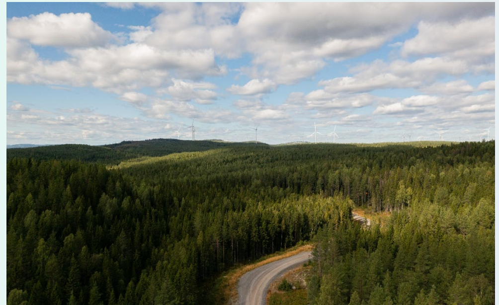
View of parts of wind park Stor-Skälsjön outside Sundsvall in Sweden. Eolus and Hydro Rein acquired and developed the project jointly. The park is now owned by Hydro Rein and MEAG. Stor-Skälsjön was put into commercial operation in 2025.
